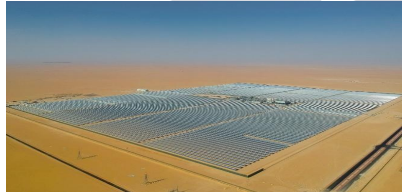
Illustration: Shagaya Renewable Energy Park (Kuwait), a vast clean energy complex in the desert about 100 km west of Kuwait City. Phase 1 of Shagaya, completed in 2018, comprises a 50 MW CSP.
